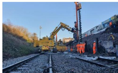
Continuous Flight Auger (CFA) on track solutions
