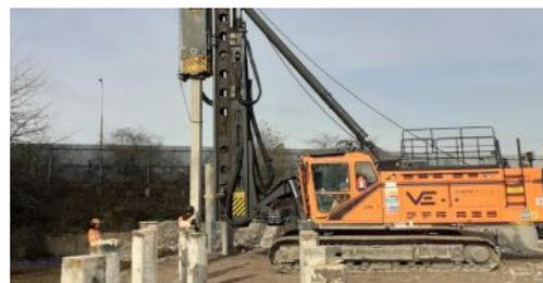
Junttan PM20 installing pre-cast driven piles
