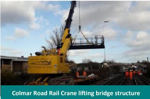
Colmar Road Rail Crane lifting bridge structure
