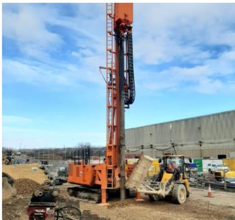
Vibro stone columns being installed in Sunderland
